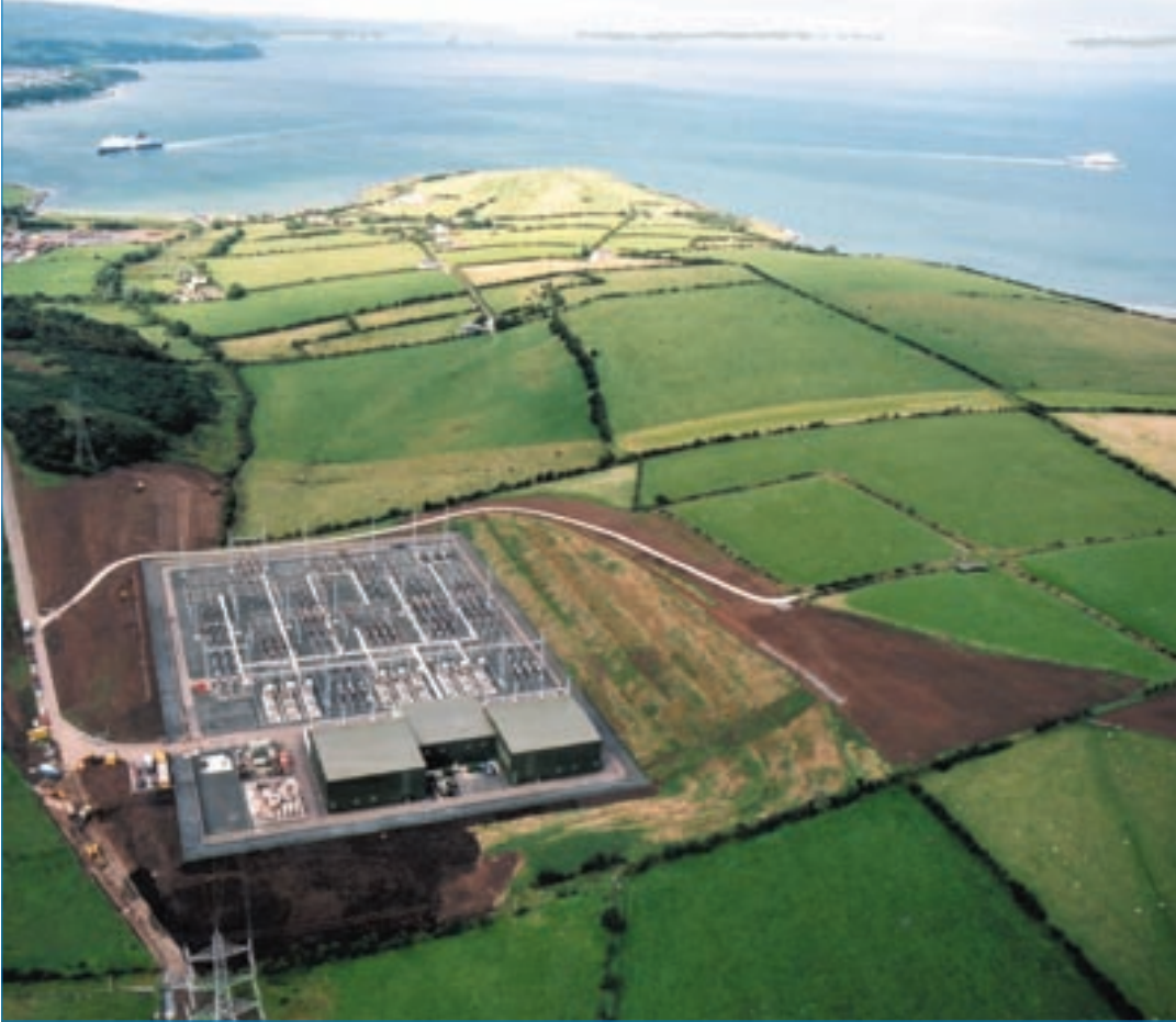
Ballycronan More converter station at Islandmagee under construction
